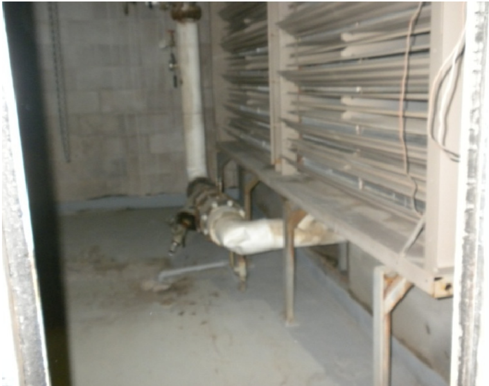
Figure 4. Old WHRS piping to the downstream side of the face and bypass damper in HVS-1.
