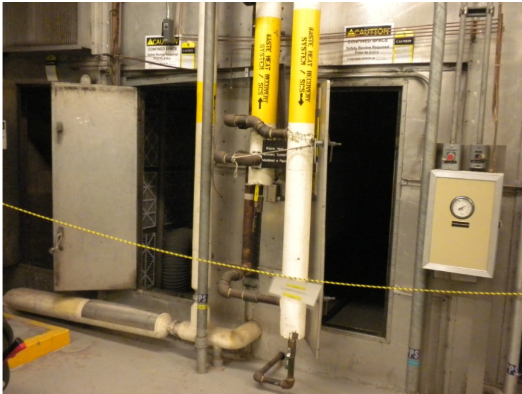
Figure 5. Old WHRS piping to HVS-5.
