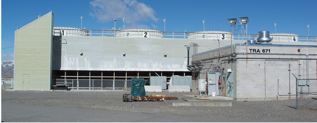
Figure 12. ATR four-cell cooling tower.
