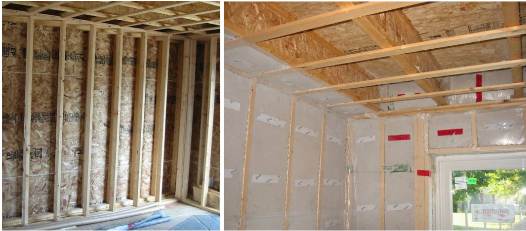
Figure 6. Double walls before and after cellulose insulation
