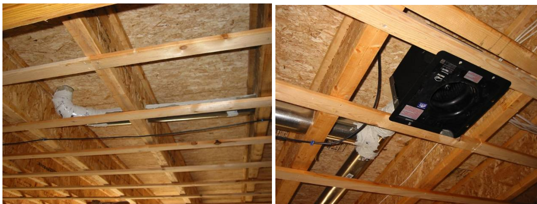
Figure 8. The exhaust fan and simple duct distribution system installed between the first and second floors
