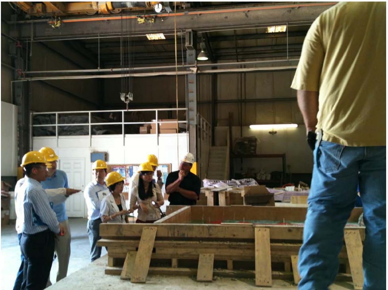
Figure 5 Viewing precast process, visible are green moisture barrier placed on top of PIR panels, connection pins, and red tape to complete the moisture barrier at these penetrations
