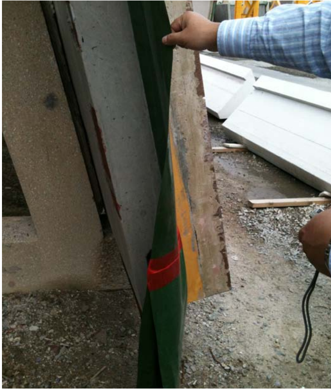
Figure 6 Cross section of insulated precast wall with integrated moisture barrier. Finished surface to the right, yellow side of polyiso layer partially visible, green moisture barrier (with red taped seam) extending out side of wall section, and plain concrete side of wall on the left
