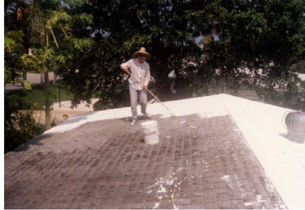
Figure 40. A highly reflective elastomeric coating was applied over shingles in an experiment in July 1992 (a practice that is no longer recommended because of moisture-related problems)
