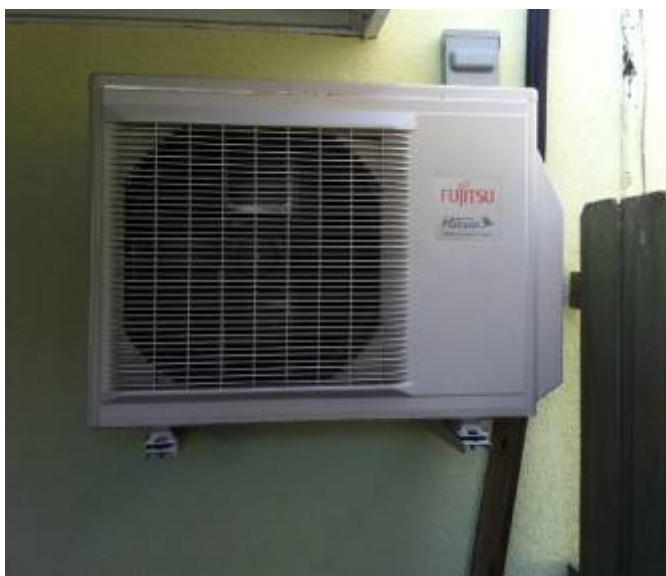
Figure 73. SEER 26 Fujitsu mini-split heat pump. The outdoor unit is located on the west garage outside face. The indoor unit is located inside the central living room, adjacent to the garage in the house.
