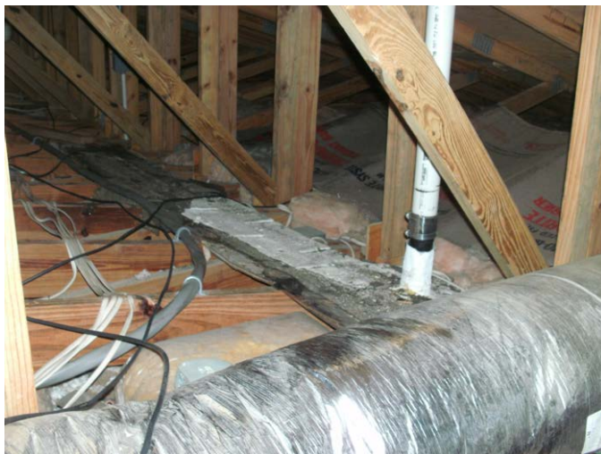
Figure 68. Attic ducts, while sealed, are only insulated to R-6 and a major source of heating system heat loss in winter and cooling season heat gain in summer. Using the mini-split allows the duct system to be largely abandoned in place without these losses for space conditioning.
