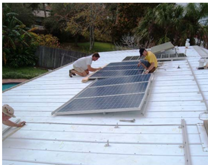
Figure 86. Installation of 4.1-kW PV system in February 2009
