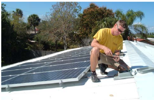
Figure ES-1. 4.9-kW rooftop PV system is connected in February 2009. The white metal roof was part of house improvements in the 1998 remodel.
