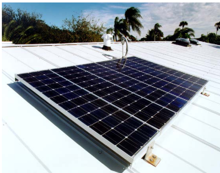
Figure 66. 450 W of solar modules powers pool pump directly. Solatube on white metal roof can be seen in the background. Array shown before installation of larger 4.9-kW PV system.
