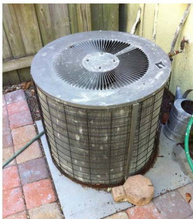
Figure 5. Outdoor unit for SEER 10, 2-ton A/C installed in 1995 and still in use
