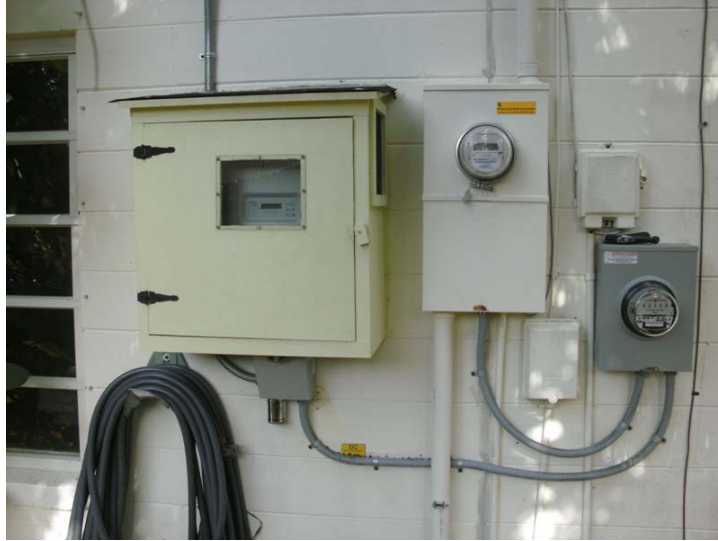
Figure 87. SMA 6000-W inverter is located on the east side of the home with the utility bidirectional meter. A ventilated enclosure was built to protect the inverter from sun and rain.
