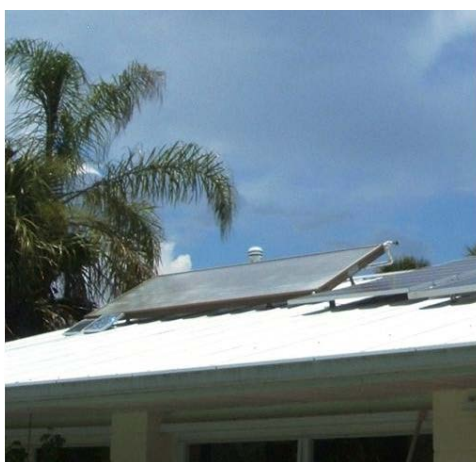
Figure 47. 4 ft × 8 ft solar collector. System is PV pumped by two 5-W PV modules mounted in parallel.
