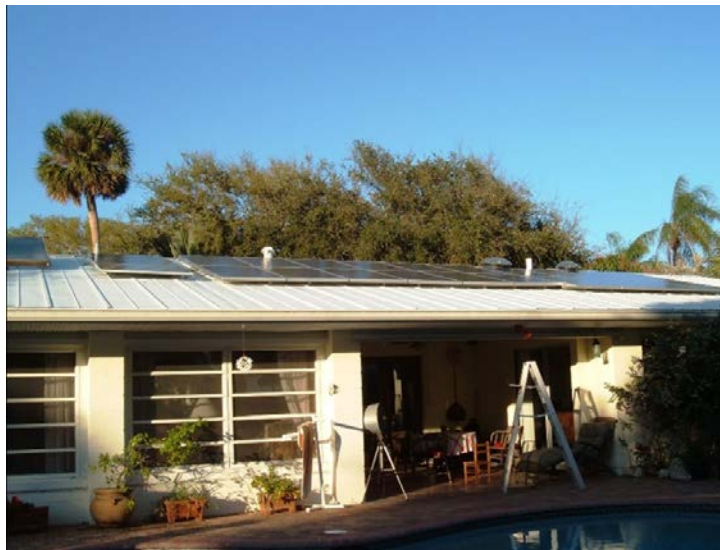
Figure 88. South roof of the home showing 4.92-kW PV system, 450-W PV pumping array, and solar water heating system (far left).
