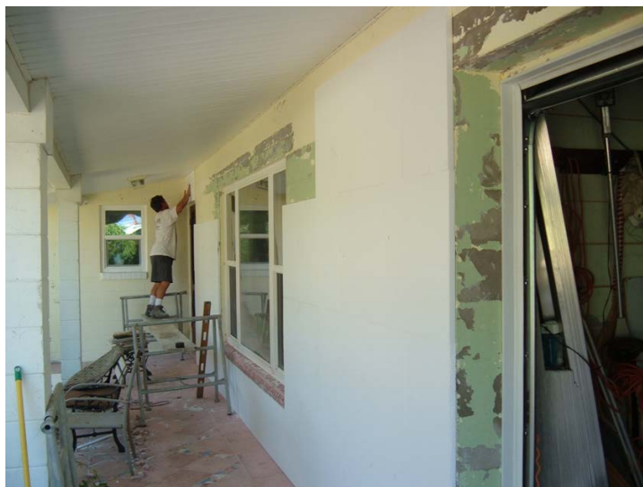
Figure 65. Exterior EIFS wall insulation retrofit in progress. Insulation consists of 1 in. of expanded polystyrene on the exterior covered by fiberglass mesh and vinyl texture stucco.
