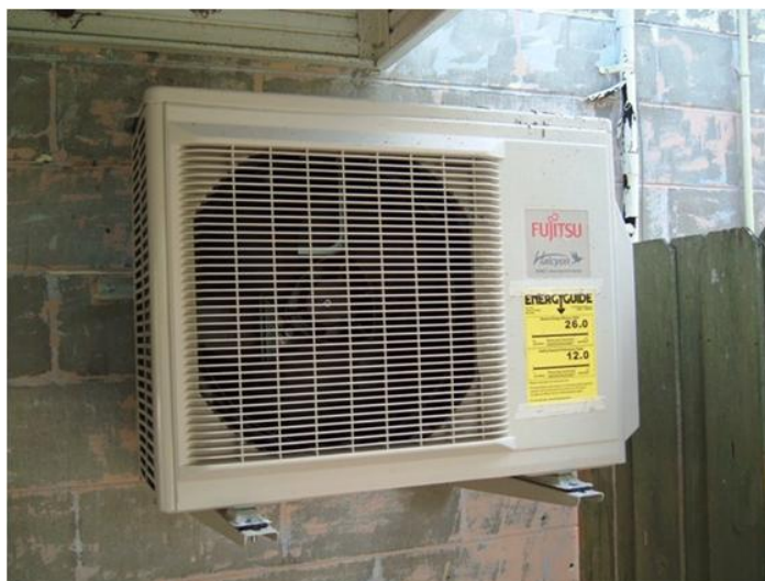
Figure 69. Outdoor unit of Fujitsu 9RLS mini-split heat pump as it appeared during the installation of the wall insulation retrofit. The outdoor unit is located outside the west garage.
