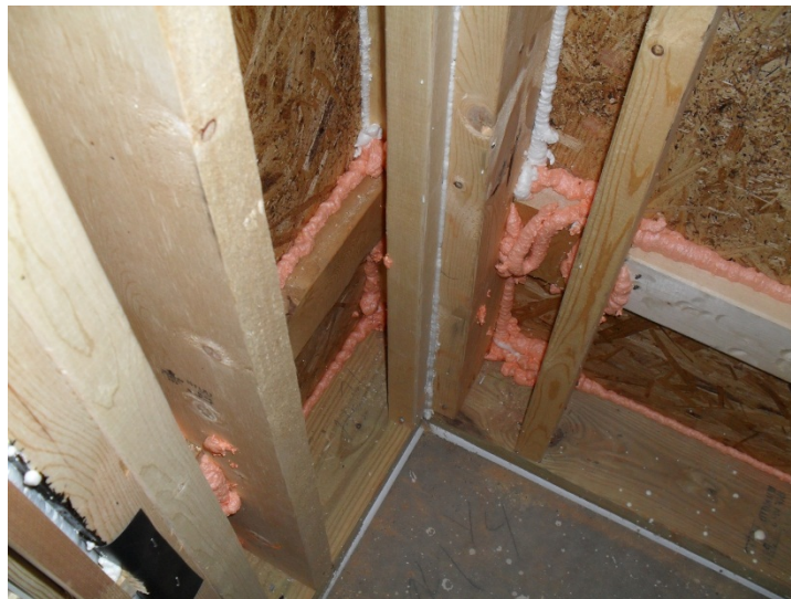
Figure 4. Air sealing detail at exterior basement wall corner, Nest Cottage nine
