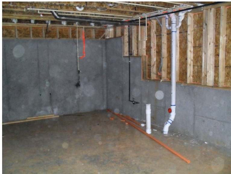
Figure 3. Foundation wall and framing, Nest Cottage nine
