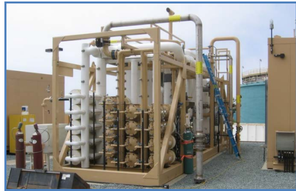
Wastewater biogas cleanup system at Pt. Loma WWTP. This privately owned and operated project processes over 1 million cubic feet of digester gas per day (which was previously flared) to generate 4.5 MW of baseload renewable power. The biogas is cleaned, injected into the San Diego Gas & Electric natural gas pipeline, and wheeled to the University of California, San Diego and the City of San Diego South Bay WWTP, which operate two fuel cell power plants to produce 2.8 MW and 1.4 MW, respectively. A third fuel cell, a 300 kW system located on site at the Pt. Loma WTP, also generates renewable power to upgrade the biogas to biomethane.
