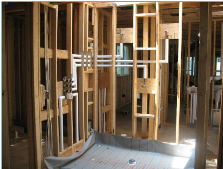
Figure 11. Insulated hot water piping at second floor shower
