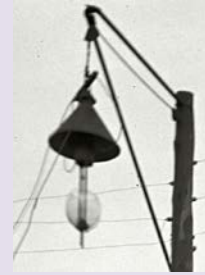
Carbon arc streetlight from early 1900s
