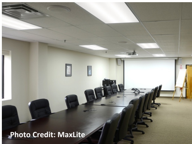
Figure 3.5 – Examples of Troffers and Other Common Fluorescent Fixtures
