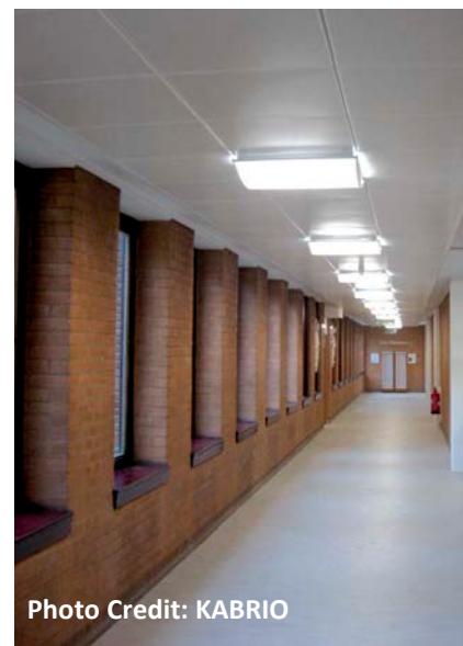
Figure 3.5 – Examples of Troffers and Other Common Fluorescent Fixtures
