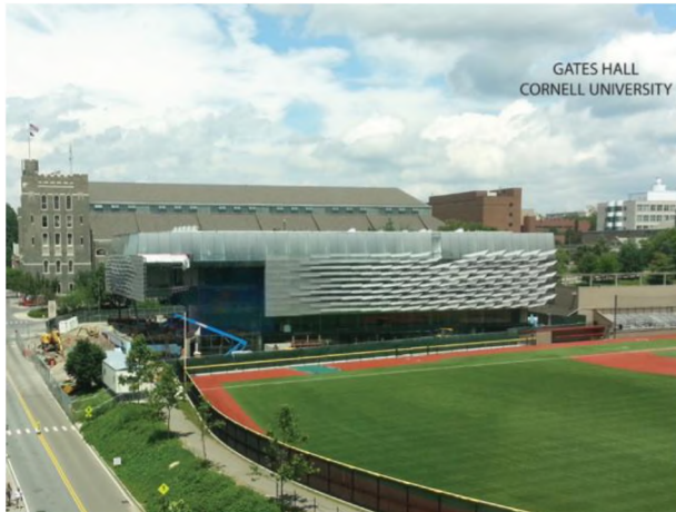
Figure 14. Gates Hall, under construction at Cornell University, (left) features perforated metal screens and fritted glass as shading devices, which was accurately modeled in SUSTAIN (right).
