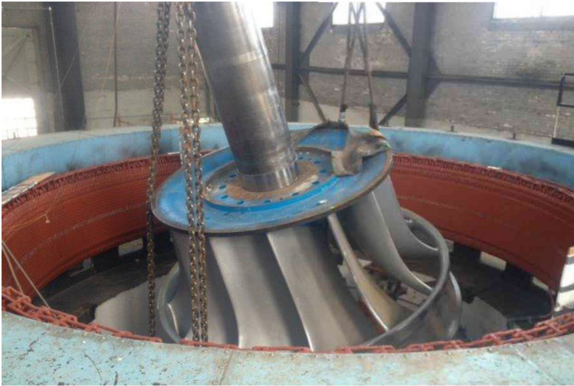
Figure 6. New Runner Installation
