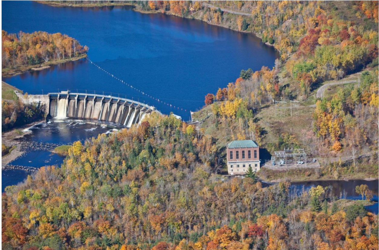
Figure 2. Fond du Lac Hydroelectric Development
