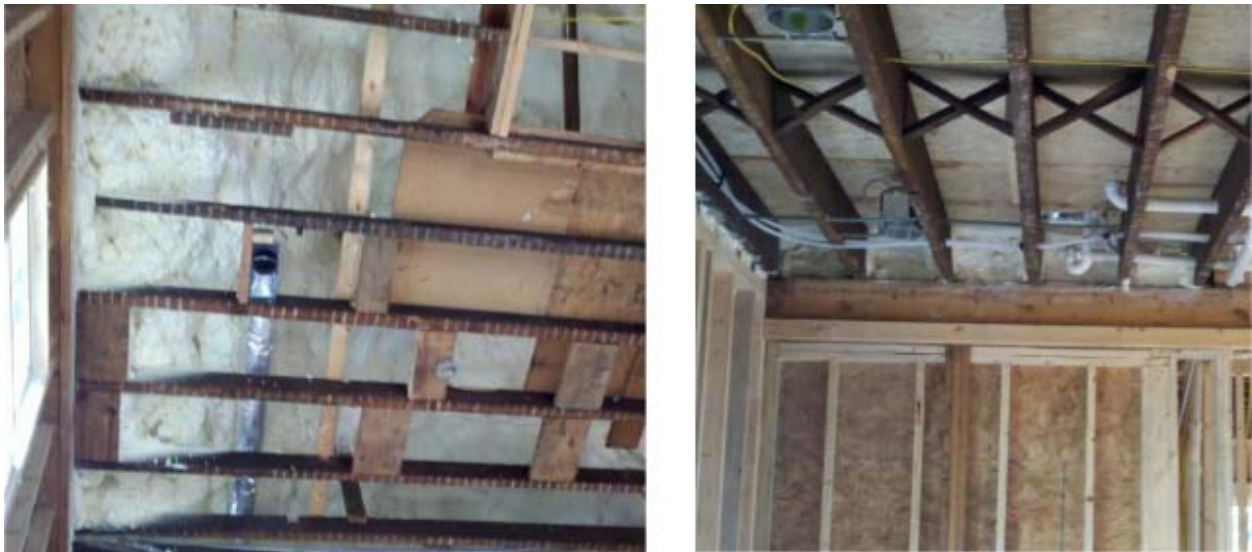
Figure 10 Left: unvented attic sealed with closed cell spray foam. Right: insulated band-joint. Images courtesy of Oak Ridge National Lab.
