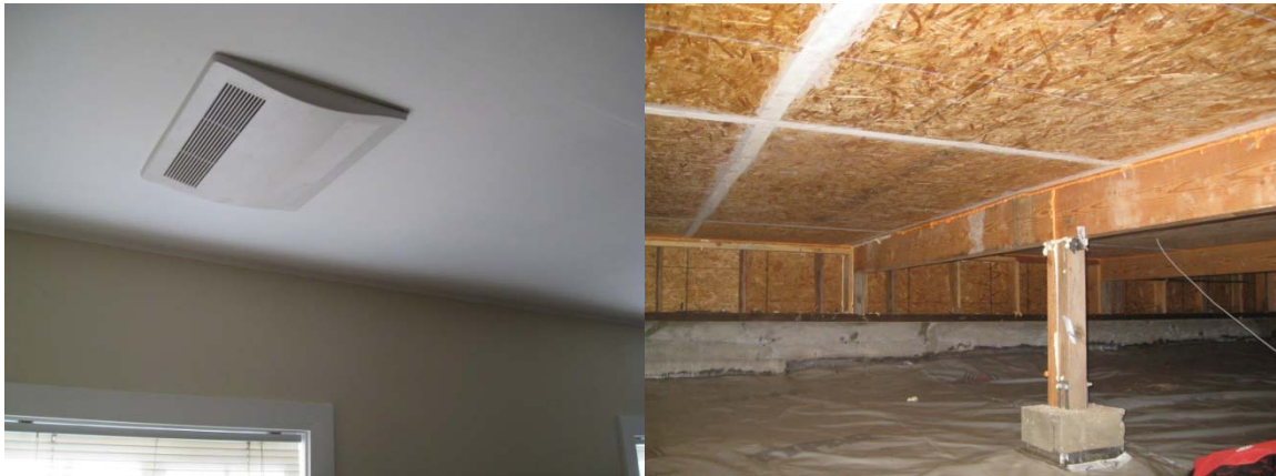
Figure 20 Left : whole house mechanical ventilation was provided by a point-source energy recovery ventilator located in the living room. No distribution was provided to other areas of the home. Right : the unvented crawlspace of the home was air sealed, insulated and water managed.
