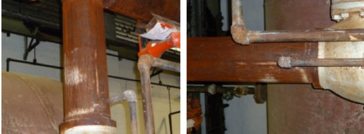
Figure 10: Target location of steam pipe for second-generation prototype at Stony Brook backup steam facility. Pipe is 8" in diameter and has a typical temperature of 350 °F.
