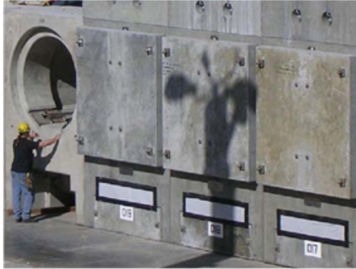
Figure 1. A photo of a horizontal dry cask storage system. 2
