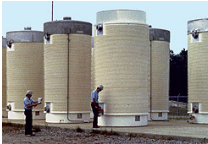
Figure 2. A photo of a vertical dry cask storage system. 2
