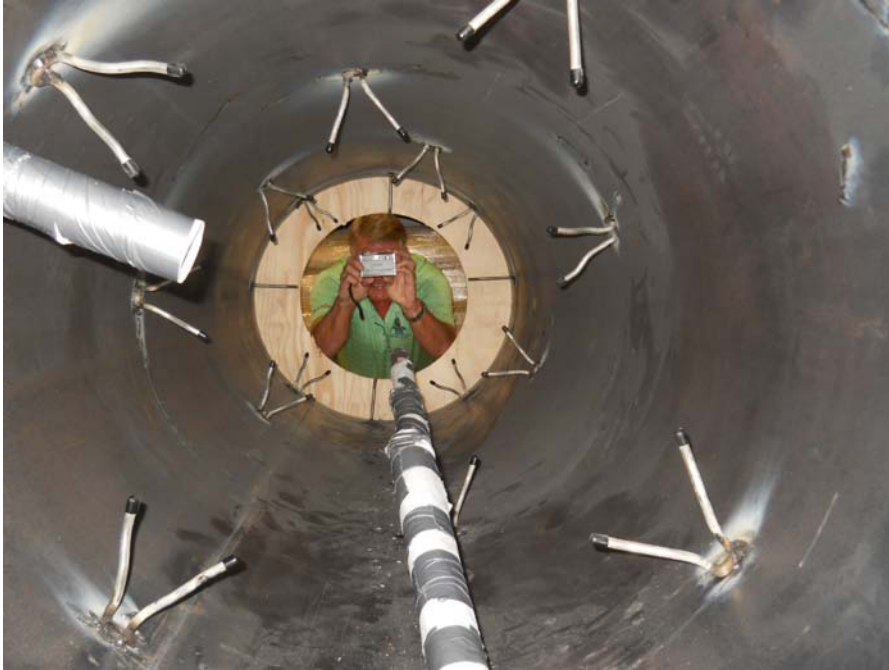
Inside Reducer Section before Refractory Installation
